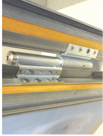
8) Hinge on fire-resistant profile
