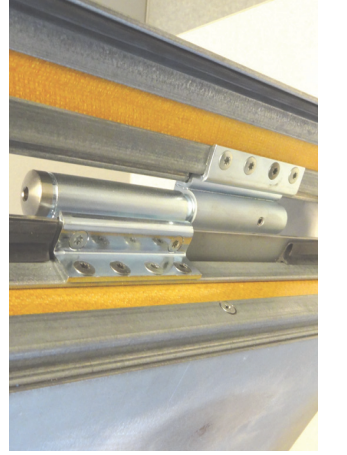
8) Hinge on fire-resistant profile
